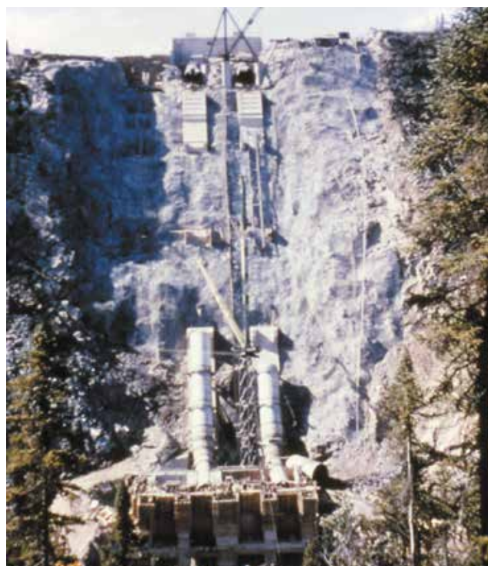
1960 Twin Falls power project under construction
